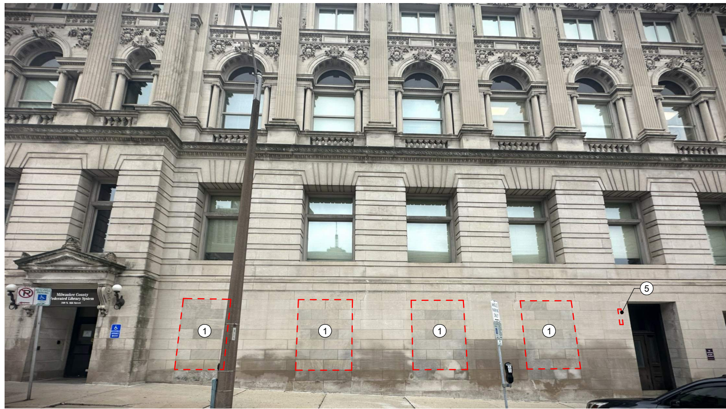
Existing Condition Photograph
